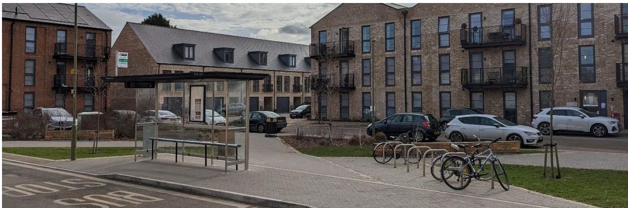
Figure 9 – Example of a suburban transport hub in a new housing development in Wolvercote
